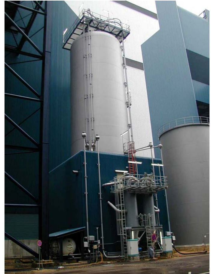
Dried Lignite Storage Silo
